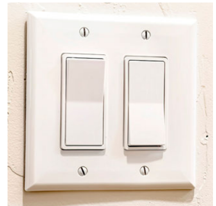
Figure 26. Flat rocker panel light switches provide greater access for workers with hand impairments.
