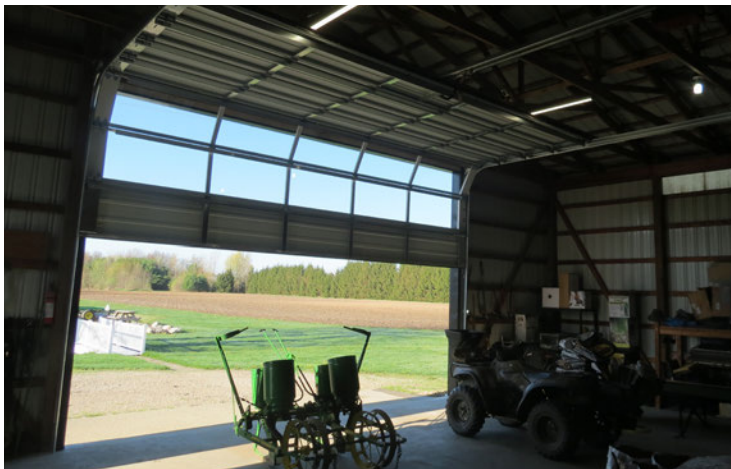
Figure 20. A segmented overhead door with windows and power opener provides natural light and remote control.
